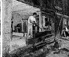
Ray works on barn
